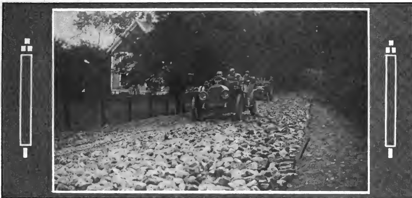
Massachusetts State Highway Encountered Before It Had Received the Finishing Touches of the Roadmaker
